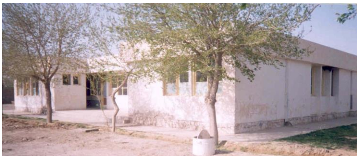
Maywand, a partially ruined MoH clinic, was rehabilitated and activated in December 1998 by AHDS. It was handed over to IbnSina in year 2002.
